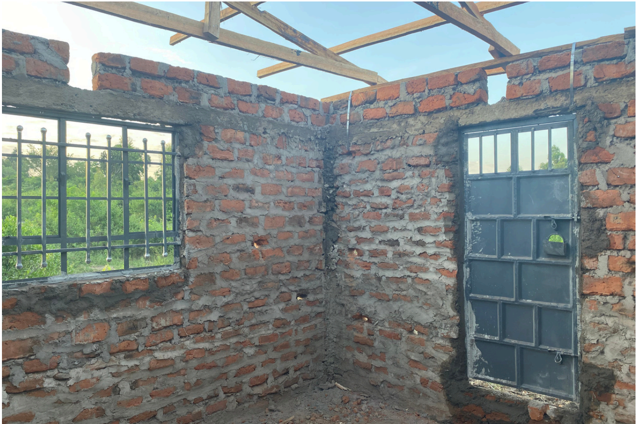
Below: Framing the roof, with windows and steel doors already installed.
