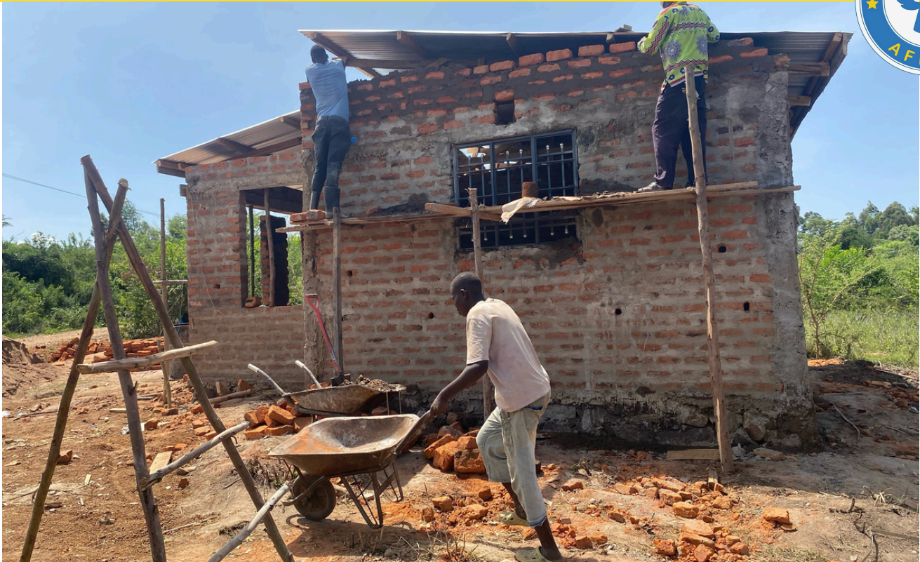
Above: Placing the iron sheets for the roof.
