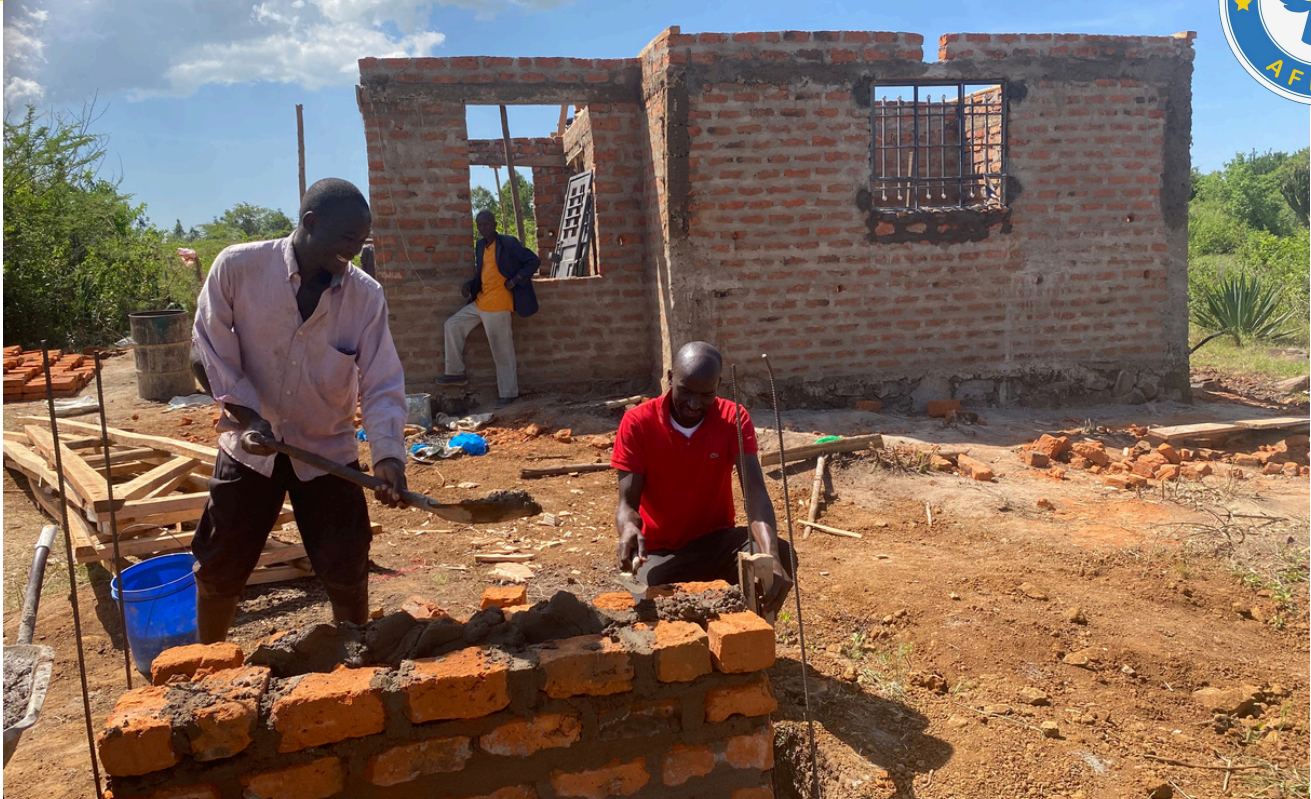
Above: Cementing bricks to build the sign.
