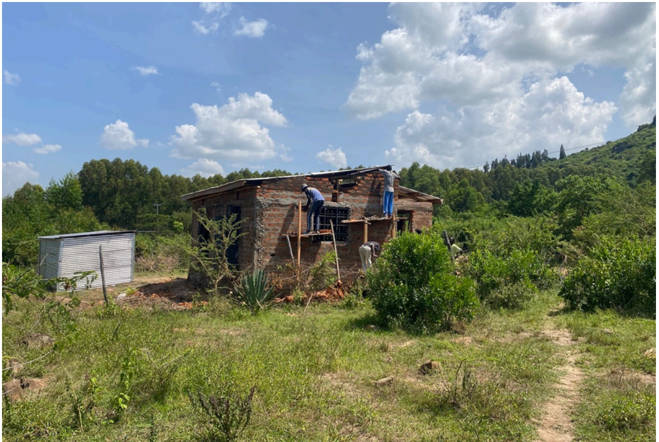
Below: Work continues sealing the walls and roof.
